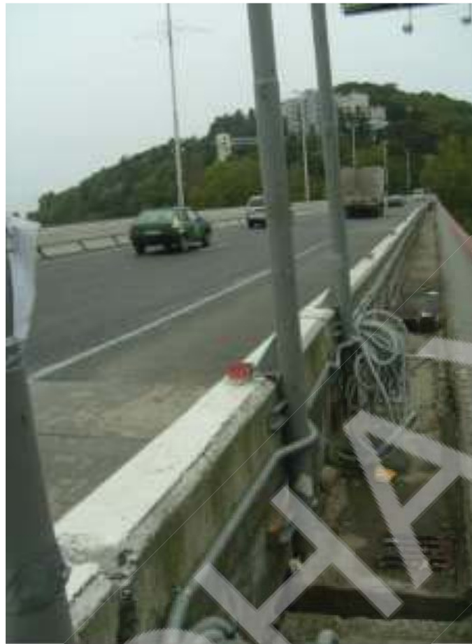
Fig. 4. Special supports to fix strain gauges-photodetectors.
