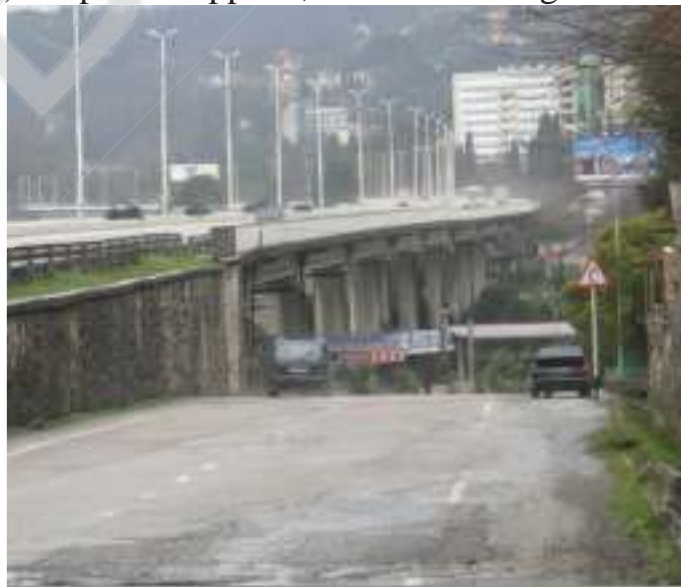
Fig. 3. Electric lighting of roadway on the bridge
