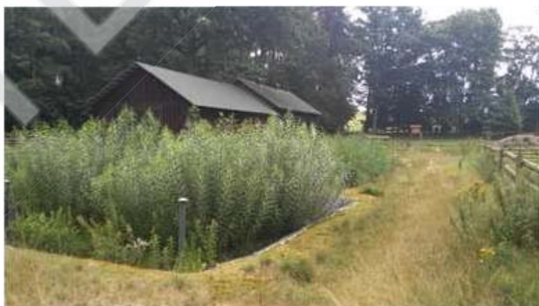
Hybrid constructed wetland in Florianka in the Roztocze National Park (VF-HF) [fot. Józwiakowska K.]
