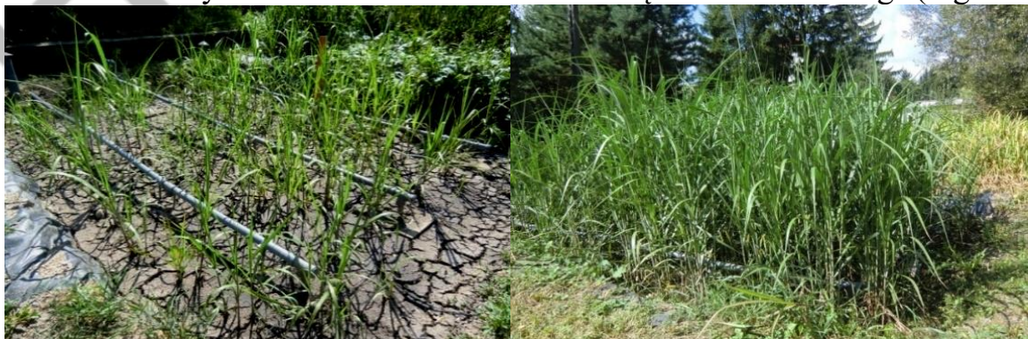
Fig.11. Constructed wetland system with common reed for sewage sludge dewatering in Dąbrowica
