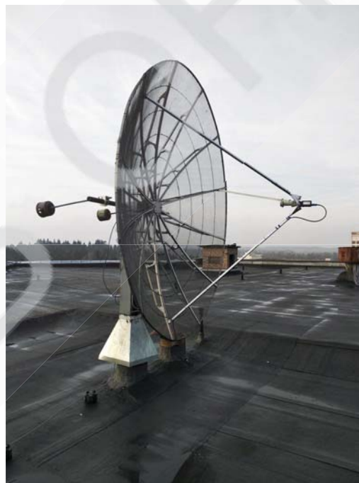
Fig. 1. Wide-aperture direct focus parabolic antenna.
